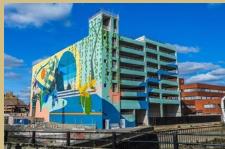
The Brentford Project Mural: artist Hixxy completed a large-scale mural on the site of a car park building, which is part of the regeneration project. The mural was commissioned for the building whilst it awaited cladding.
